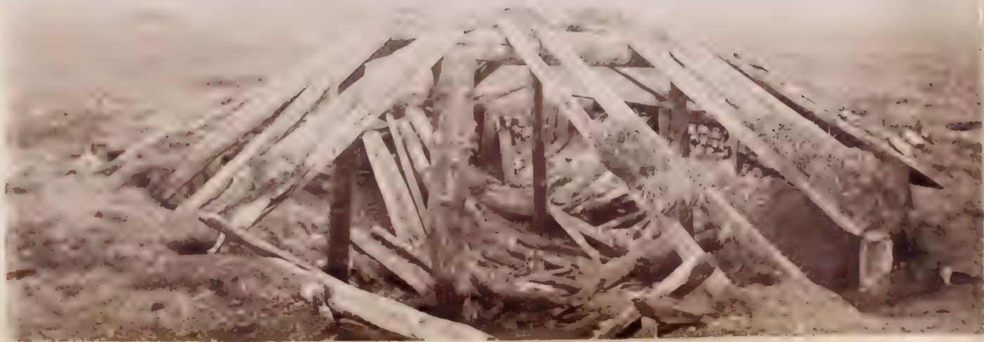
Ruined house, Pt. Lawrence Island, June, '95.
